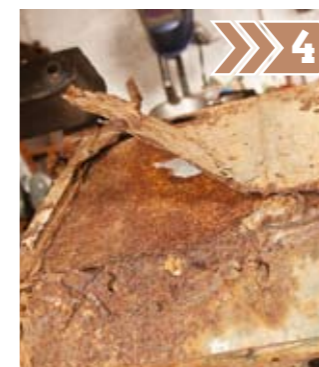
4 ...but the original rotten metal was left underneath the patch and has now ‘blown’ away from the repair.
