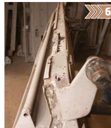
6 The top rail is often badly rotted. Water collects under the windscreen and is trapped by the sealing rubber. This one’s been hidden by paint, but is a relatively easy repair...
