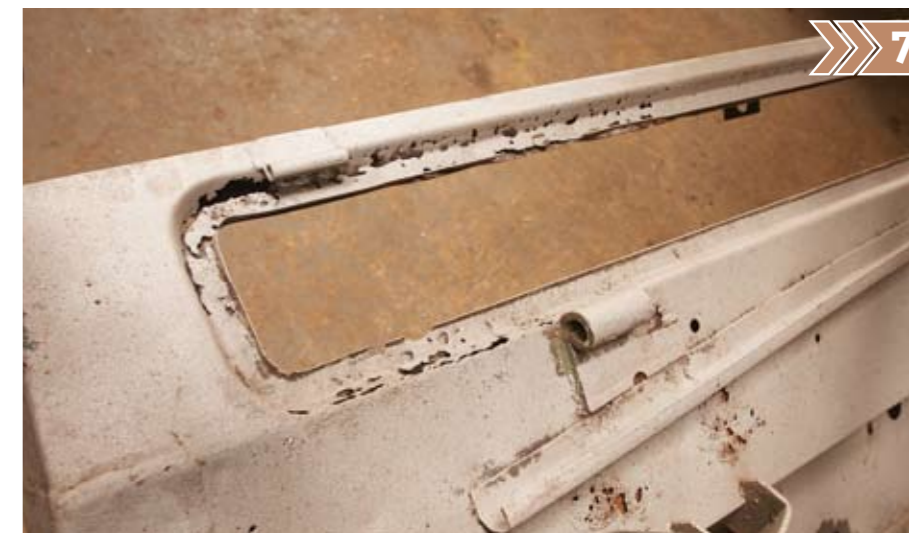
7 ...Unlike the area around the vent flaps. ‘This really isn’t a job for the faint-hearted’, says Kev. ‘It will take as long to repair this section as it will to replace a footwell and door pillar. The really bad ones are put to one side and done on a ‘as and when’ basis.’
